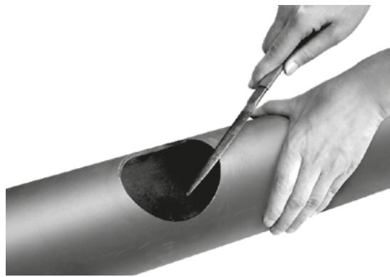
**Remove beads and rough edges** and clean the pipe surface within a radius of 16 mm around the hole in which the gasket is to be seated. This area should be checked to ensure a clean, smooth surface, with no recesses or protrusions that could affect the quality of the seal. The area within the "A" dimension should also be checked for dirt, scale or any defects that could affect the effective seating of the gasket or the assembly of the coupling.
