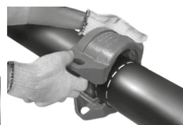
**Install casing elements:** Place the casing components around the gasket, making sure that it is centred between the first marks drawn at the pipe ends on the inside and that the casing elements are centred between the second markings drawn on the outside. Make also sure that the feather and groove of the casing are aligned.
