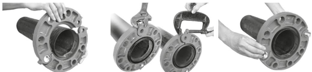
**Install the articulated flange structure (2-12"):** Open the articulated flange structure. Place the flange segments around the groove at the end of the pipe and tighten them together until the bolt holes are aligned.
