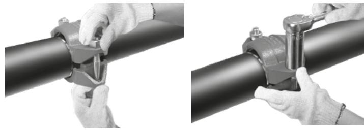
**Insert the bolts and put on the nuts:**
