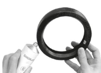
**Lubricate the gasket:** To facilitate insertion of the pipe and installation of coupling without pinching effect, apply a thin layer of KAN-therm grease on the lip of the gasket and on the outer coating of the gasket. Other suitable lubricants may be used as long as they do not have properties that may damage the gasket. In systems exposed to extremely high or low temperatures, it is recommended to use a silicone grease.
