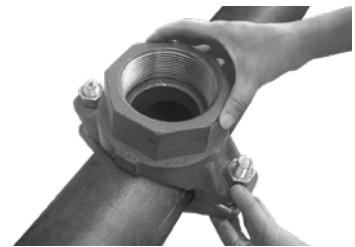
**Check the retaining flange:** Make sure that the retaining flange is properly seated in the hole. You can check this by swinging the top of the casing in the hole. Make sure also that the oval bolt head is locked in the bolt hole in the coupling casing.
