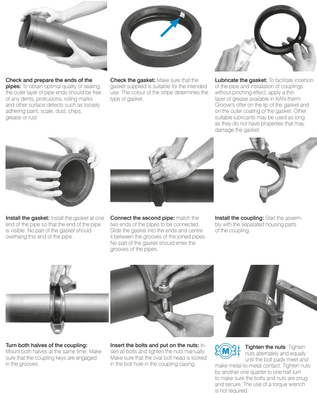
**Check and prepare the ends of the pipes:** To obtain optimal quality of sealing, the outer layer of pipe ends should be free of any dents, protrusions, rolling marks and other surface defects such as loosely adhering paint, scale, dust, chips, grease or rust.
