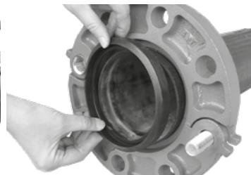
**Install the gasket:** Place the gasket in the recess between the outside diameter of the pipe and the recess in the flange. Make sure that the lower part of the gasket (marking side) is positioned and seated on the bottom of the gasket pocket.
